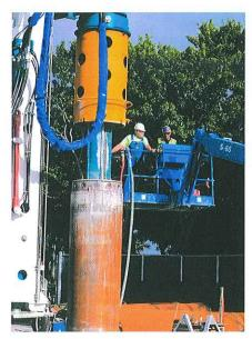
plished without damaging or impacting the existing FM located with an invert about 20 ft below mudline because it had to remain in service. Once completed, the retrieval shaft was 13 ft in diameter.
