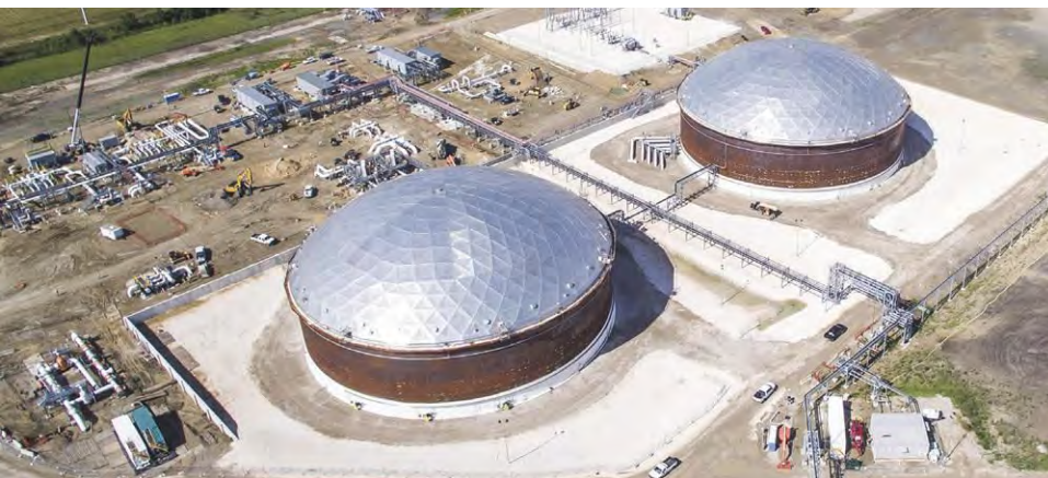
Last year at TransCanada Corp.'s crude oil tank terminal in Houston, a new interconnect system was installed. Key components include one mainline pump, two 350,000 oil-barrel tanks, and two 2,000-horsepower booster can pumps.
