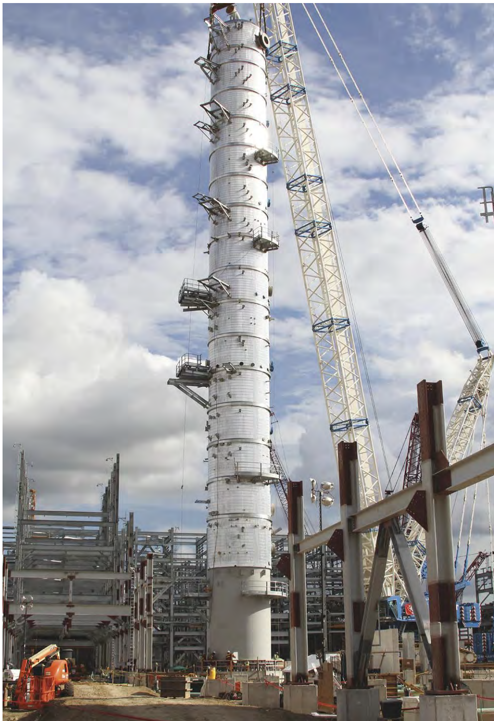
Chevron Phillips Chemical Co. is developing a 1.5-million-metric-tons-per-year ethane cracker at its existing Cedar Bayou complex in Baytown, Texas. Shown here is the 250-ft-tall, 570-ton C2 Splitter used for olefin separation.
