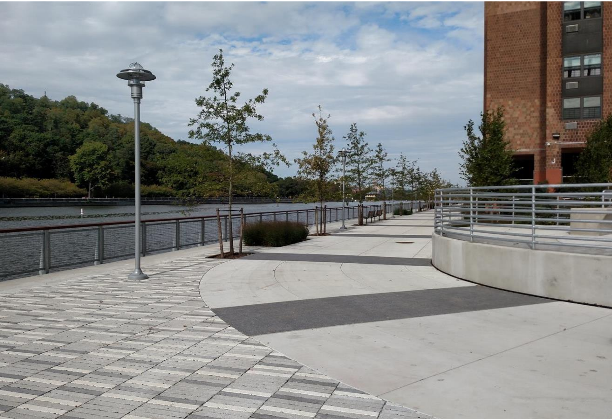
Roberto Clemente State Park, Harlem River Esplanade, Bronx, NY View Looking North of Southern Approach with South Plaza Overlook Visible at Right
