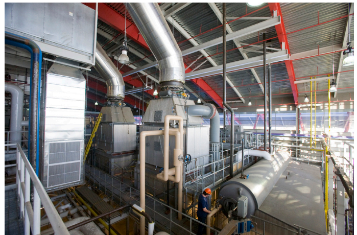
University of Massachusetts Amherst Central Plant
