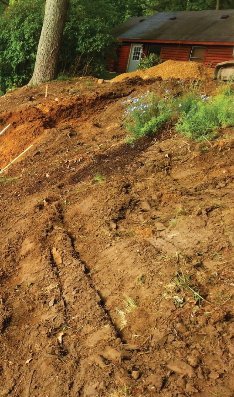
The slope being cleared and prepared for construction
