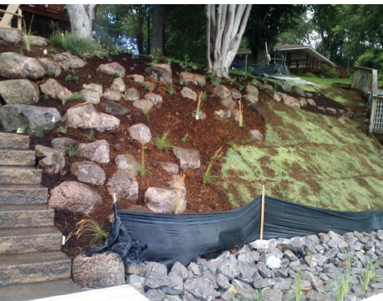
The immediate post-construction slope with the pre-vegetated blankets, boulders, and native plants
