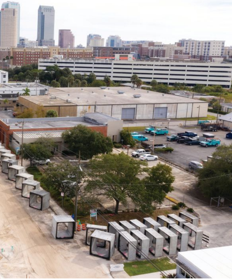
The Cypress Street Outfall project during construction.
