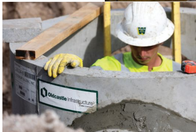
Installation of Oldcastle's custom stormwater infrastructure
