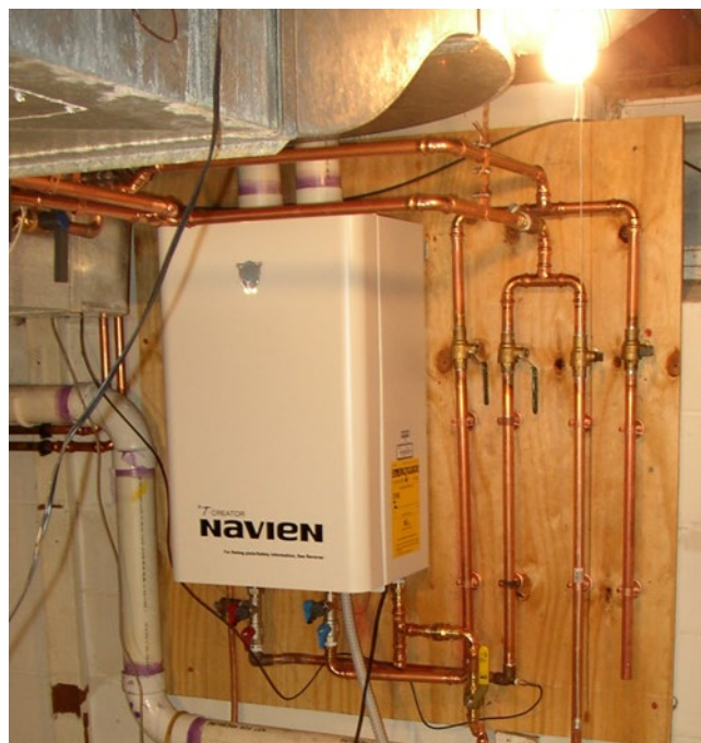
Figure 33. Example of a tankless water heater
