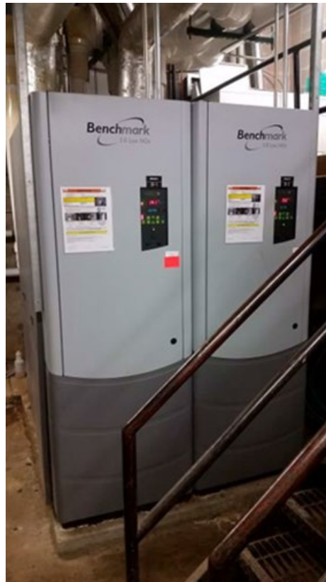
Figure 35. Example of a condensing boiler in a commercial application.
