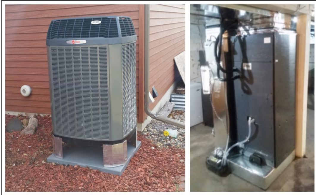
Figure 27. Example of installed cold climate central air-source heat pump
